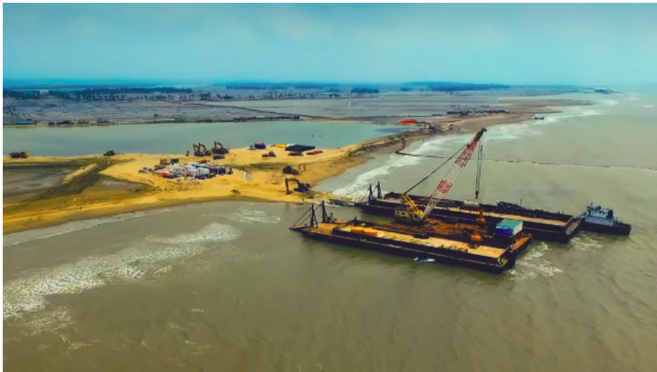
Construction work begins for the Japanese-financed Matabari Power Plant, Bangladesh (CPGCBL)
